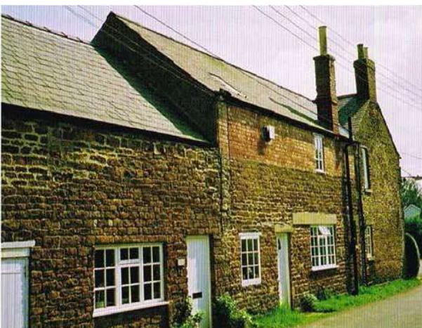
Figure 5.5b: Side view of Old Vicarage on Church St.
