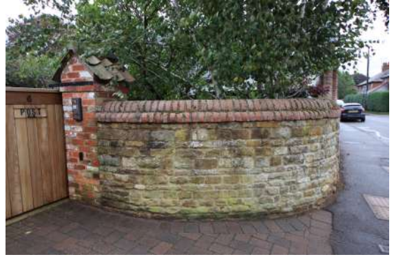
Figure 5.6: Yew Tree House entrance on Burley Rd
