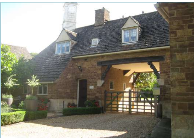
Figure 2.2: Grade II listed Gatehouse to Old Hall.
