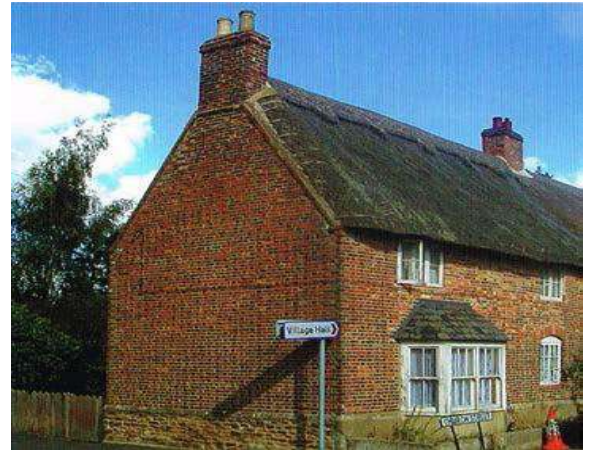
Figure 5.3: Flemish Bond on Church St.
