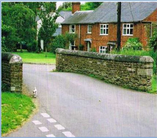
Figure 8.10: Bridges on Bridge Street (top) and Church St.
